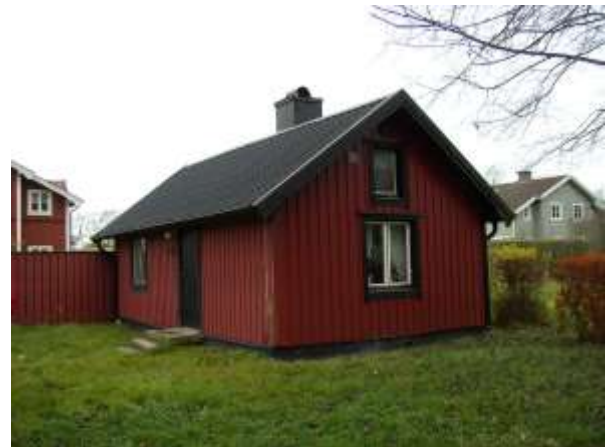
Home to Emma, 3 brothers, 1 sister, and her parents. The house has had a new roof and siding put on, but it's still the same size. Now it's used for a summer vacation house.
